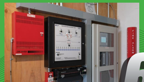
ICS-Integrated Communication Systems Wires Fire Alarm System At Design Tech High School
