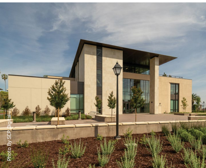
Sprig Electric installed 12 KV switchgear with 480/277V and 208/120V power, which was distributed throughout the building.
