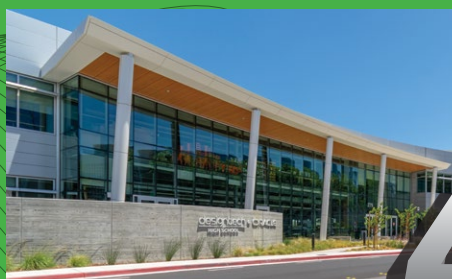
Intrepid Electronic Systems & TDN Electric Install Turnkey Emergency Responder Radio Coverage System For Design Tech High School
